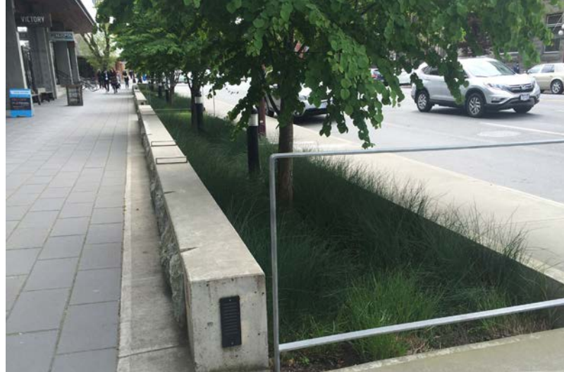
A stormwater swale in a downtown street
