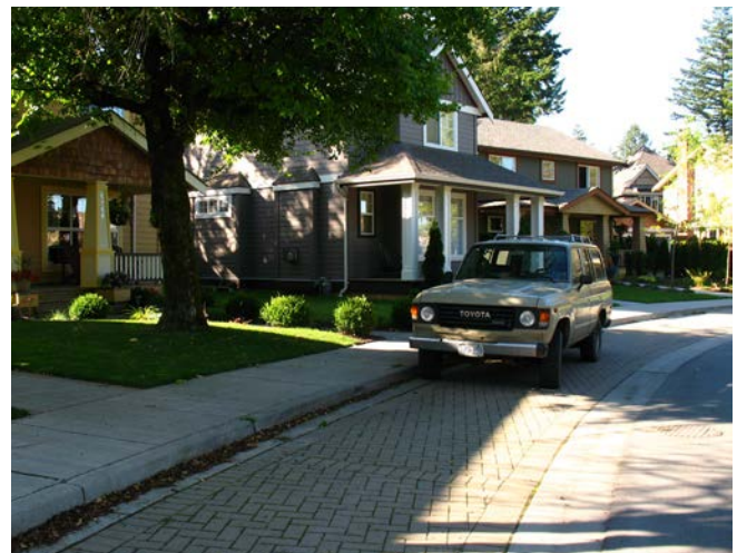
EXAMPLE: On-street parking using decorative pervious pavers, providing both attractive design and rainwater management.
