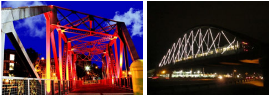
Figure 14 Gateway Improvement Examples – Cowichan River Bridge Lighting
