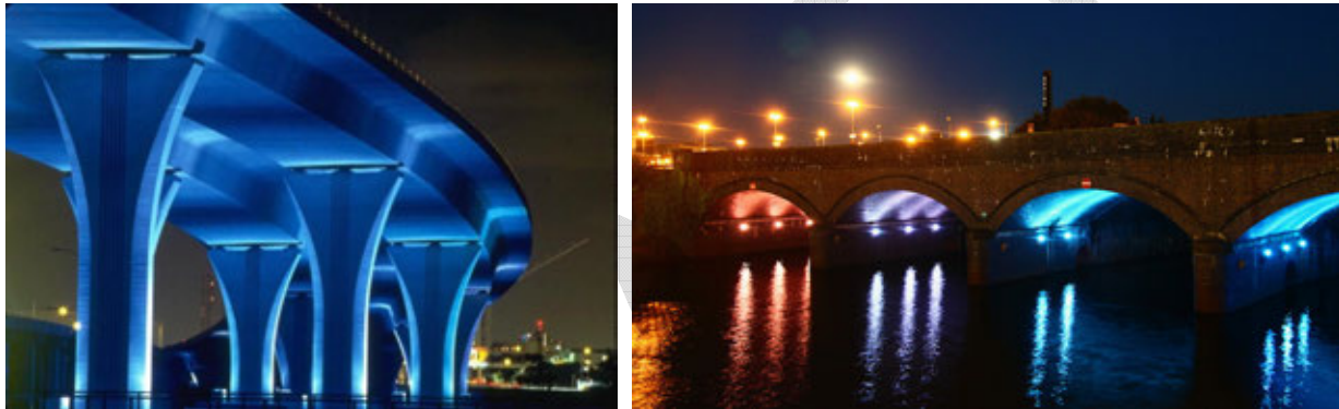
Figure 25 Pathway Safety Lighting Under Cowichan River Bridges Examples
